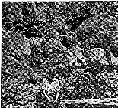
The exposed sand face on the side of the work chamber (before concrete lining was placed). Note bedding planes, stratification and lack of horizontal uniformity. The sand is brownish from oil, which oozes out in some places and sometimes trickles down the sand face.
