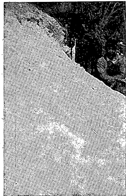
One of the piles of sand washed by gravity from a shot horizontal well. More than 250 barrels washed out in 2 shifts. No piece of rock was found larger than a pinhead.
